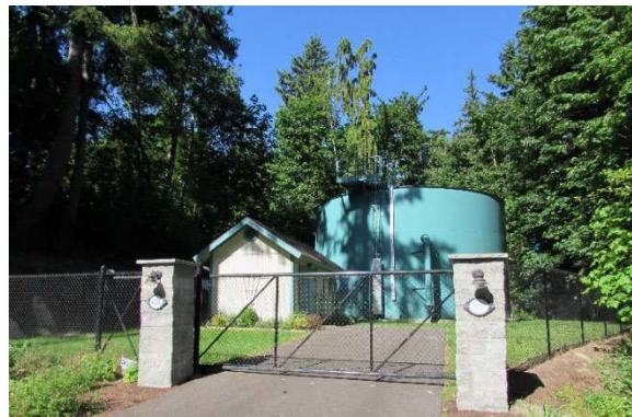
Banner Road Tank and Booster Pump Station
