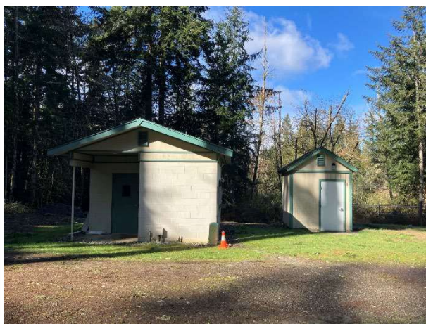
Well 5R Building & Treatment Building
