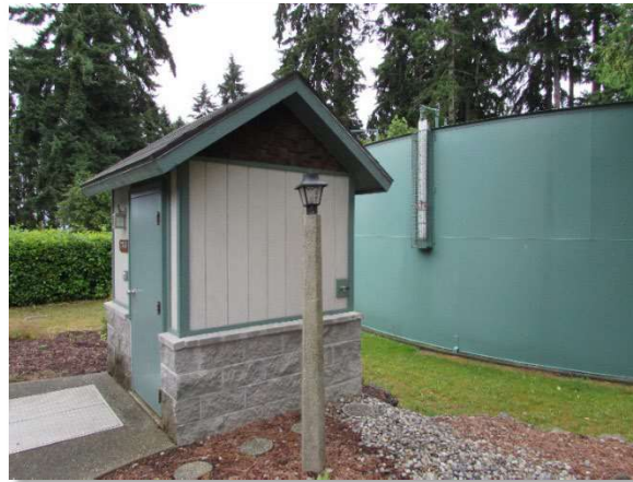
Cedar Avenue Tank and SCADA Building
