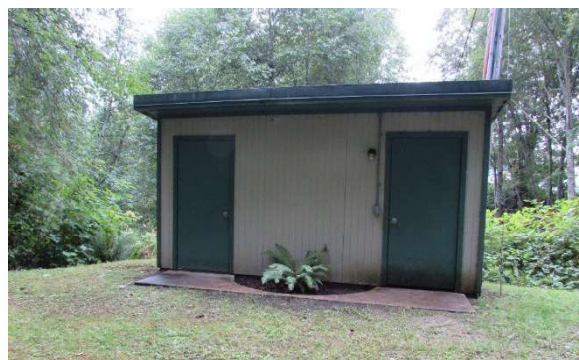
Well 2 Chemical Feed and SCADA Building
