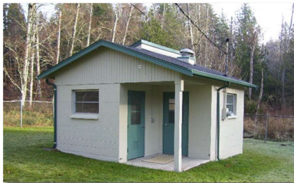
Well 4 Pump Room
