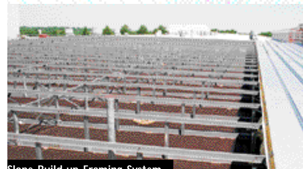
Slope Build-up Framing System
