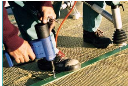
left: clips installed on the fixing rails right: expanding rivets are used to fix the rails in position
