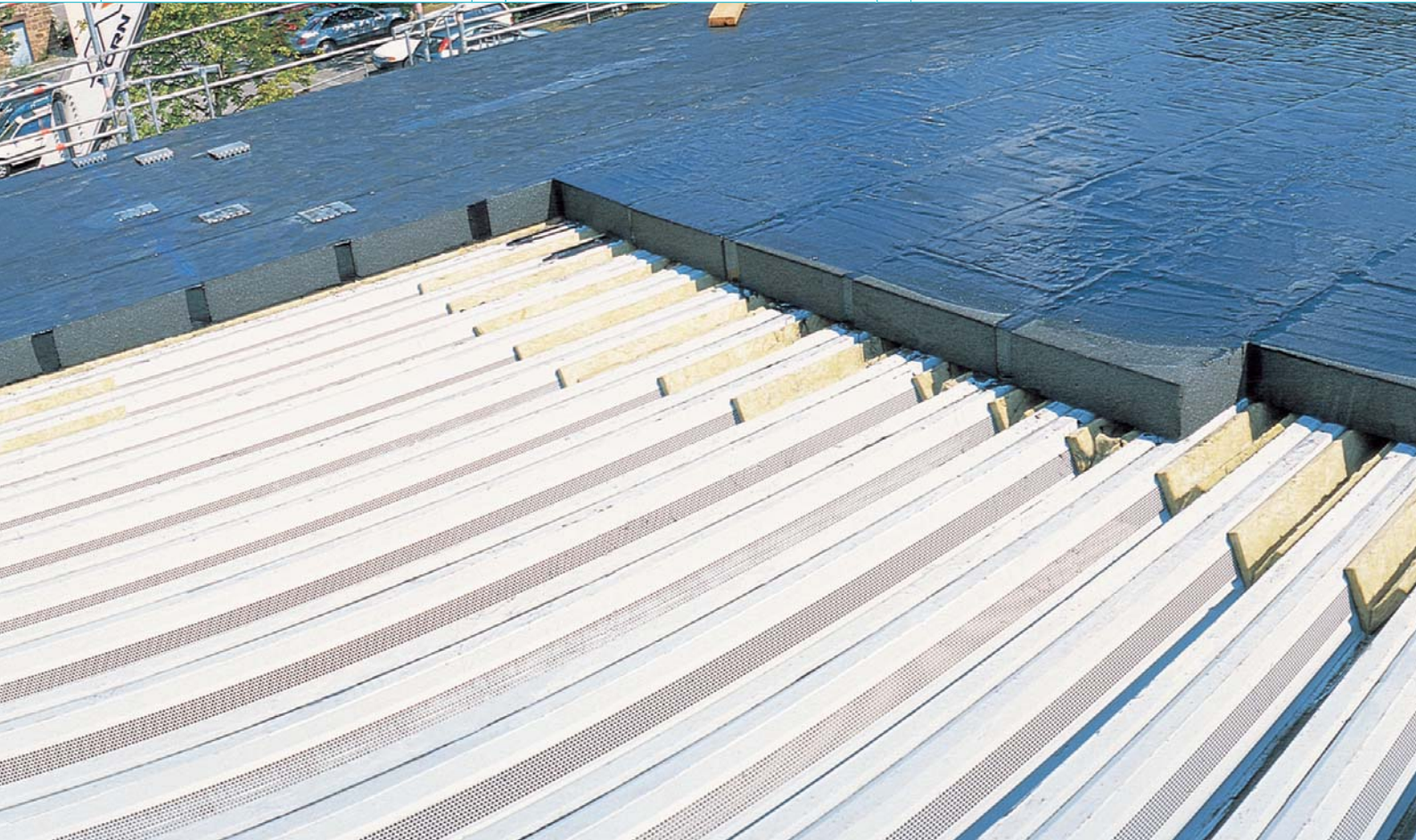
below: Perforated trapezoidal profile on a sports hall roof with soundproofing inserts. The Foamglas slabs are bonded to the upper flange using a cold bitumen adhesive; the butt joint is sealed in the edge dipping process and then coated with hot bitumen.
