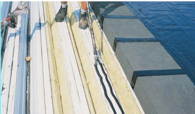
The insulating slabs are cold bonded to the substructure
