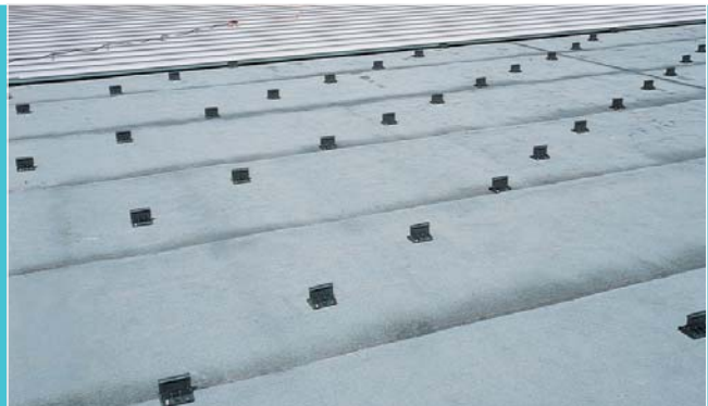
Kalzip compound clips on L-shaped claw plates with secondary sealing
