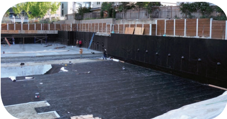
Underseal® waterproofing system utilized for entire foundation. Underslab (horizontal) installed with tie-in to Blindside (vertical).
