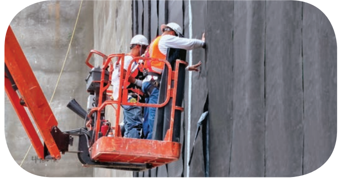
Blindside™ Membrane installed for areas requiring waterproofing that cannot be accessed from the positive side.
