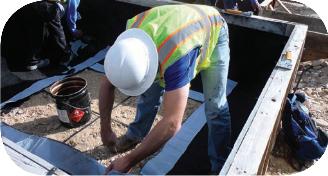
Underlab Membrane being installed to waterproof an elevator pit.
