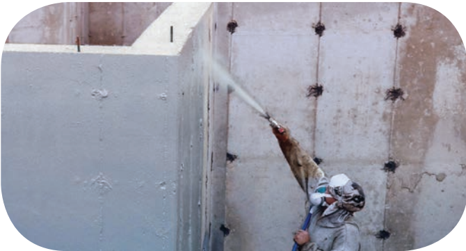
Commercial Stretch Fluid-Applied Waterproofing being installed on a foundation wall.
