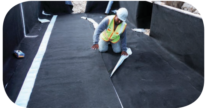
The self-adhering side laps make installation of the Underseal® Underlab Membrane quick and efficient.
