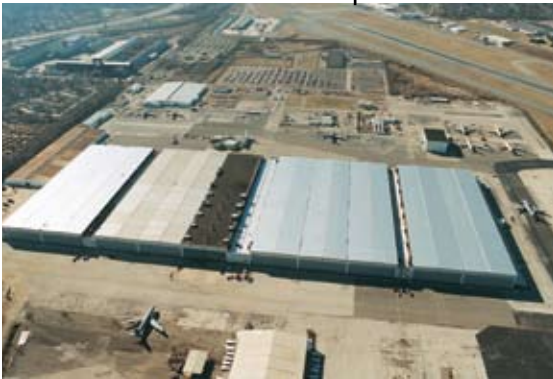
Each of the 10 connected hangars making up the massive facility can hold five to six planes the size of a Boeing 737.
