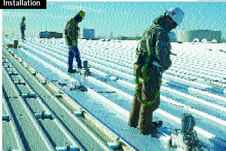
Install a retrofit MR-24 roof system over an aged metal roof while your business goes uninterrupted.
