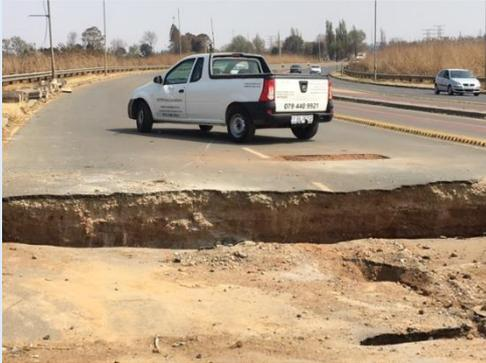
We provide dolomite stability investigations to eliminate the risk of building on such land. The study commences with a gravity survey. The purpose of conducting the gravity survey is to measure the earth’s gravitational field and then use the contrast between low density overburden and high-density bedrock to construct a contour map. This map is used to estimate the depth of the bedrock from the surface. The gravity map is then used as an aid in selecting the drilling points.
