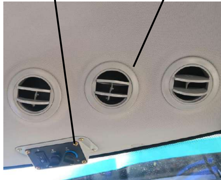
Air conditioner Switches Air conditioner Vents
