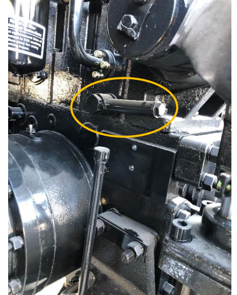
Drain Hydraulic ISO46 Oil Here
