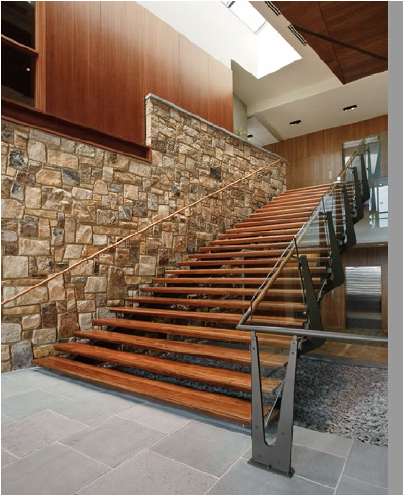
Luck Stone Staircase and Railing with Yeager Design/Fabrication Walnut, Painted Steel and Glass
