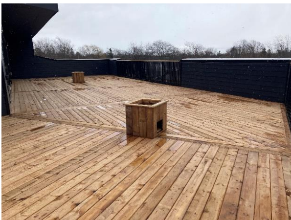
Rooftop Patio at 27 Wright Cres.
