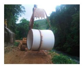
Kier Construction Company Ltd -2013-6.3 MW Maggotty Hydro Expansion Project - Installation of the New Black River Pipe Bridge
