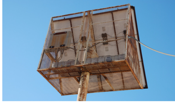
A good example of how not to build a solar power system.
