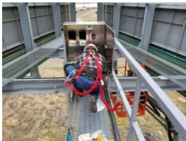
Working on the controls.
