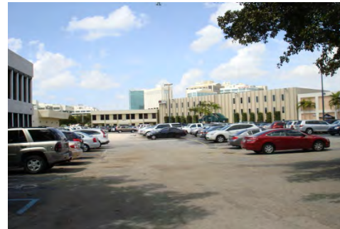
Existing Rear Connection to Parking Lot
