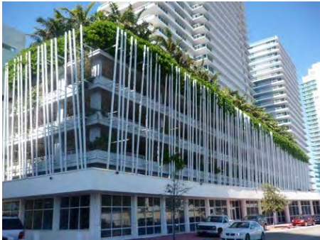
Screened Parking Garage
