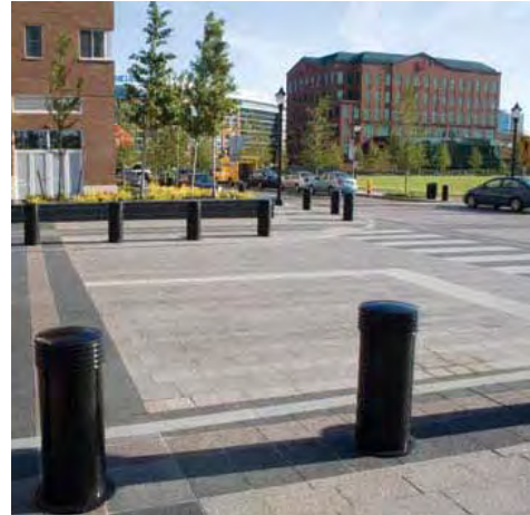
Unique Crosswalk Markings
