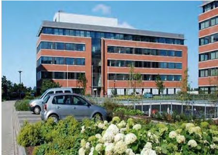
Rooftop Parking Lot with Direct Access
