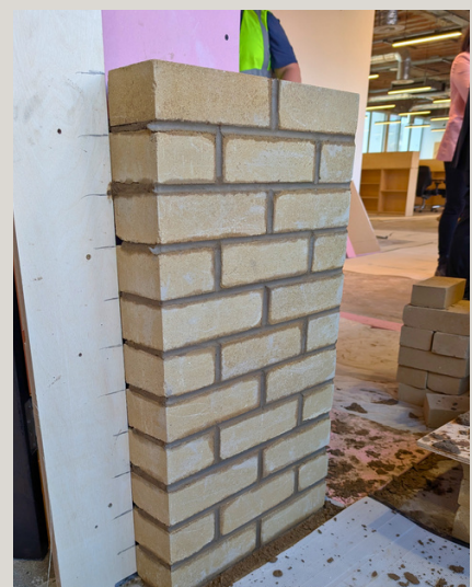
Work in progress in Manchester
