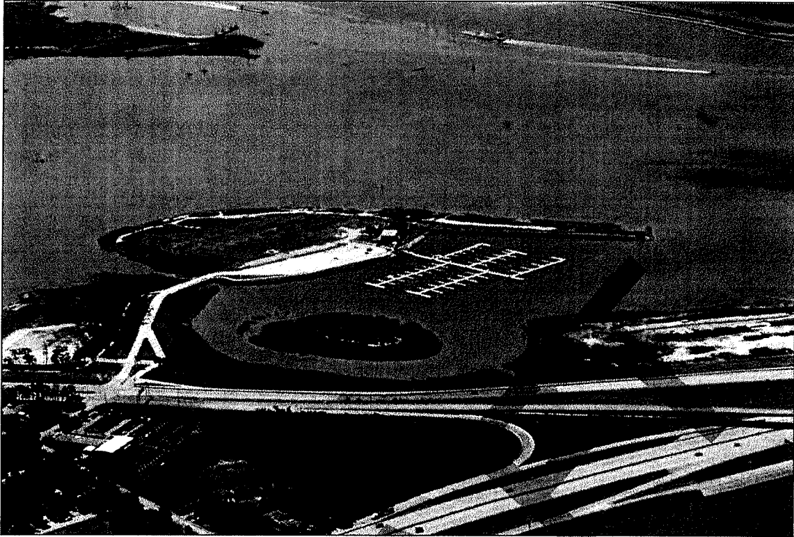
Arial View of Subject Site on Bayland Island
