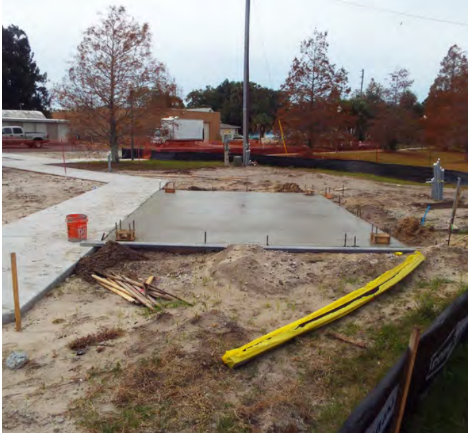
TANGERINE GREENWAY - TROLLEY MARKET SQUARE CONSTRUCTION IN PROGRESS
