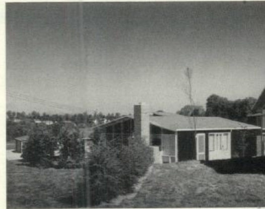
Small lots, averaging about 60' x 125', and lack of big trees called for considerable ingenuity in siting. Some privacy is achieved by angling the houses; and some by use of planting-screens, good-sized pines grouped in front of living room window-walls. To add home variety and interest, the cypress siding walls are painted dark red, yellow or brown.
