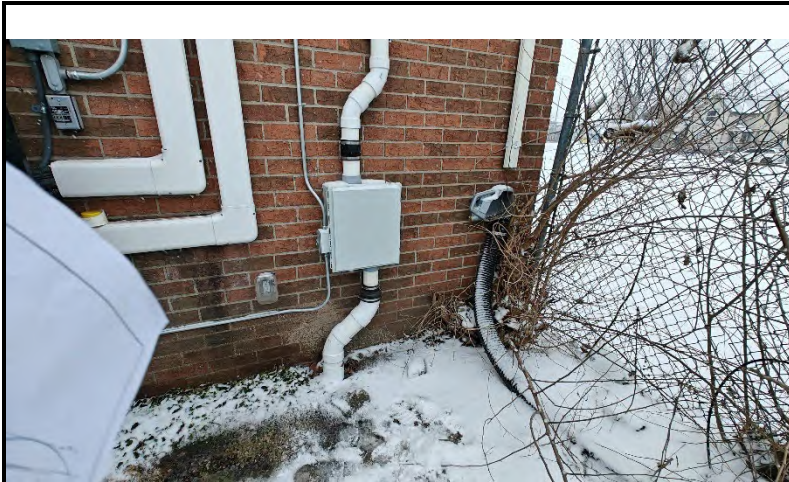
16. Representative view of OBAR fan (Fan I) and vertical vent piping.
