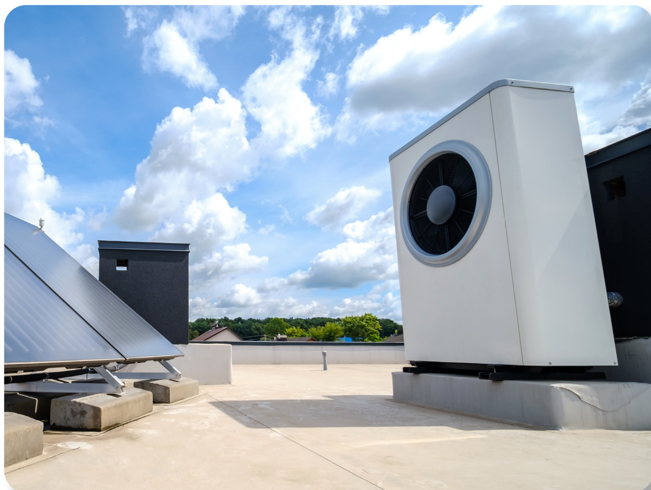
Figure A9: Heat pump and solar collector on roof of a building.
