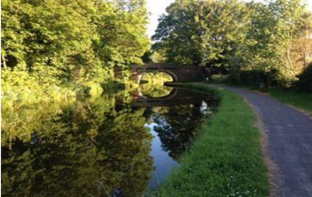
Photo 4. Hatlex Bridge (No. 119) on Lancaster Canal
