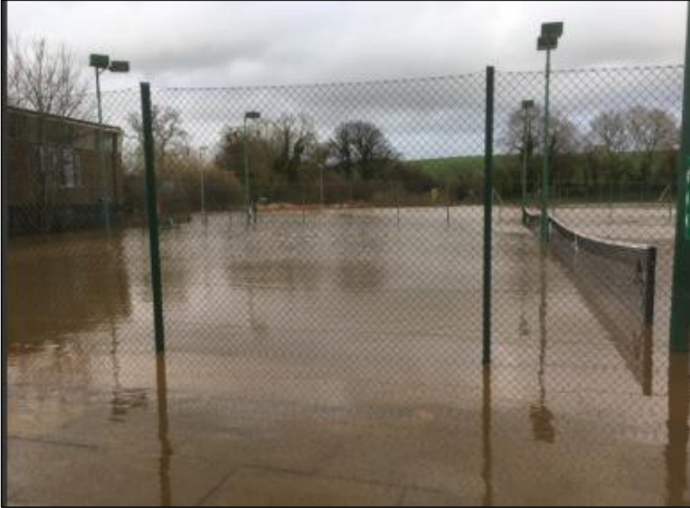
Photo 28. Flooding of Tennis Courts at the Recreation Ground
