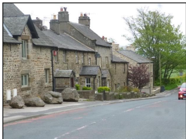
Photo 6. Stone Cottage, Main Road, Slyne
