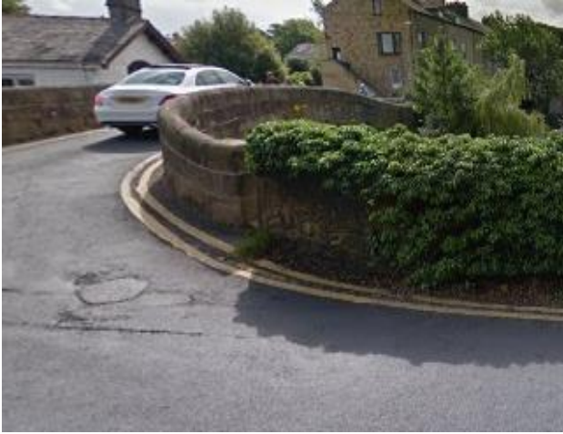
Photo 33. Canal Bridge on Hest Bank Lane
