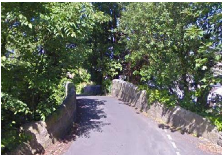
Photo 34. Canal Bridge on Hatlex
