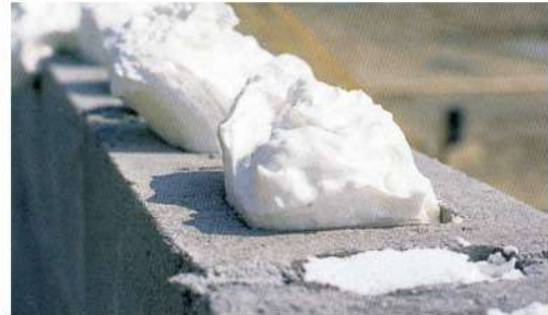
Tailored Foam Block Wall Insulation
