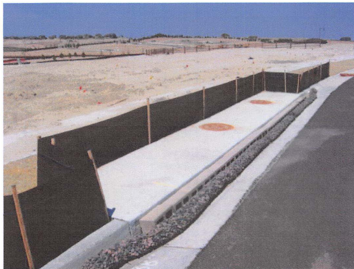
Photograph IP-1. Inlet protection for a curb opening inlet.
