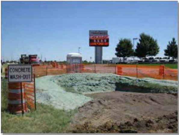
Photograph CWA-3. Earthen concrete washout. Photo courtesy of CDO1.
