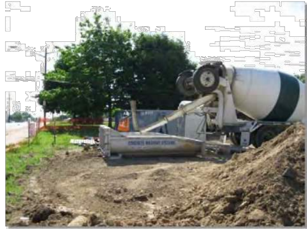
Photograph CWA-2. Prefabricated concrete washout. Photo courtesy of CDO1.
