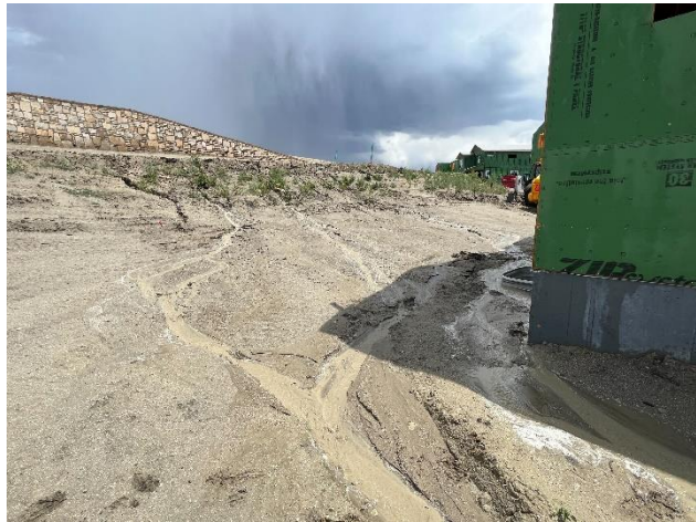
Description: WATER FLOWING OFF HILL TO EINDOW WELLS
