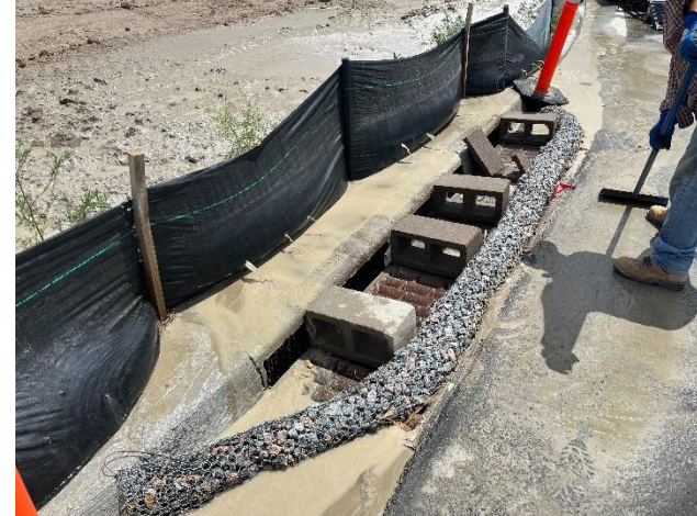
Description: SECOND INLET BEING CLEANED.
