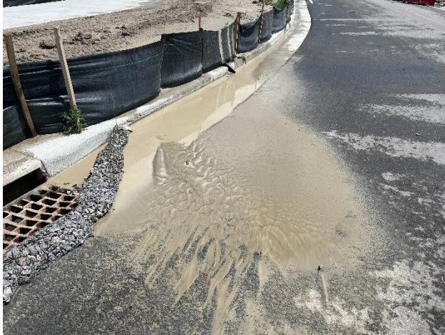
Description: SEDIMENTATION AT FIRST INLET
