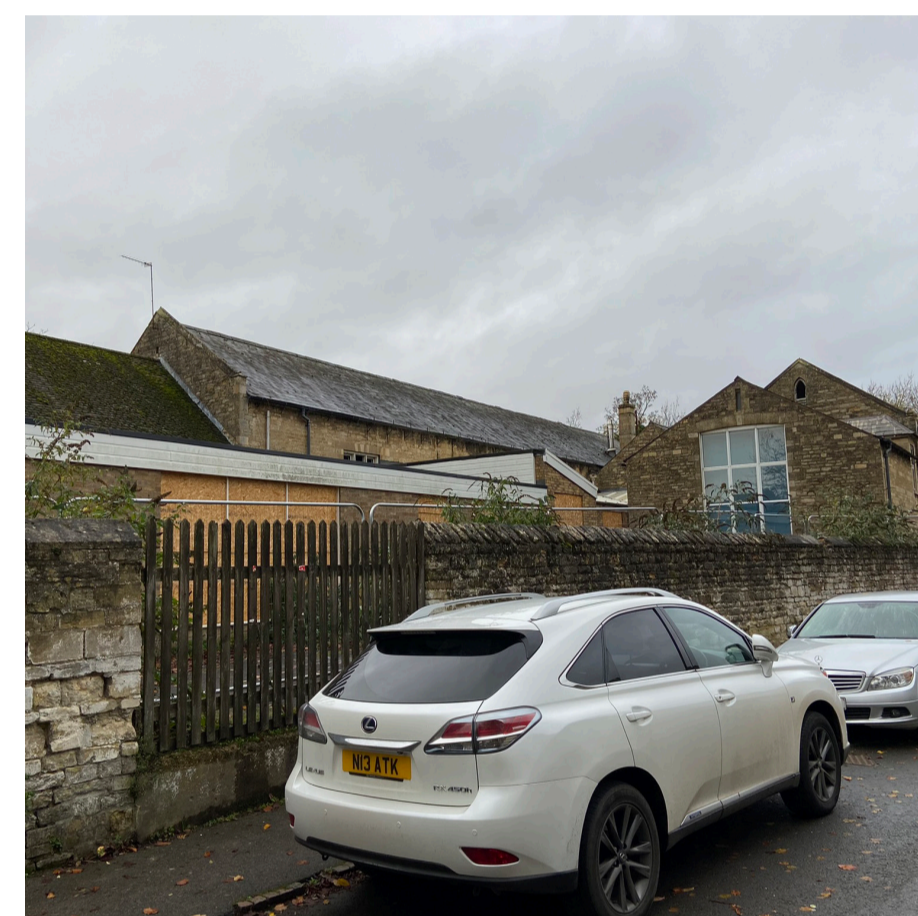
View 4 - Drumming Well Lane view showing the unattractive roofscape & elevations.
