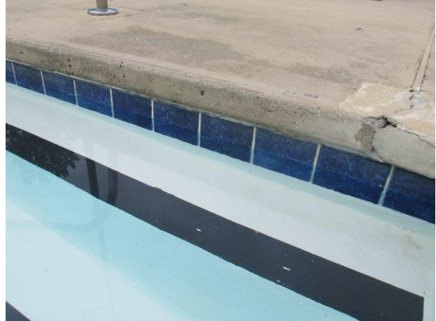
Plaster and tile at pool perimeter
