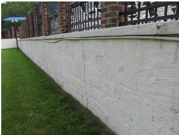
Retaining wall at pool deck – cracks evident
