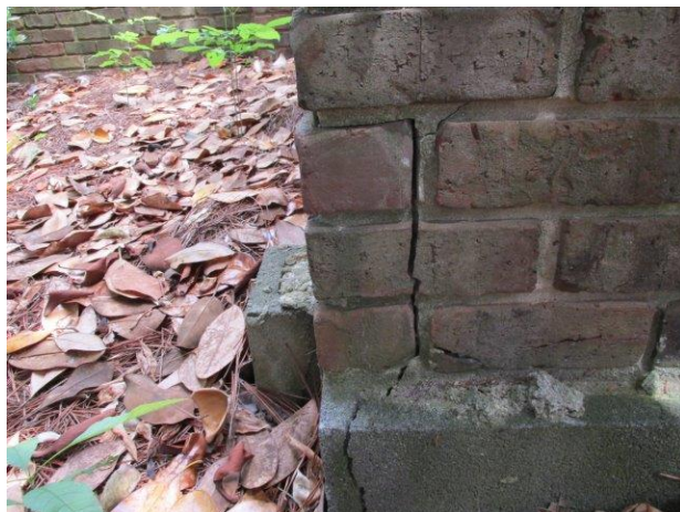
Cracks at masonry evident
