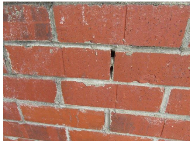
Example of mortar deterioration
