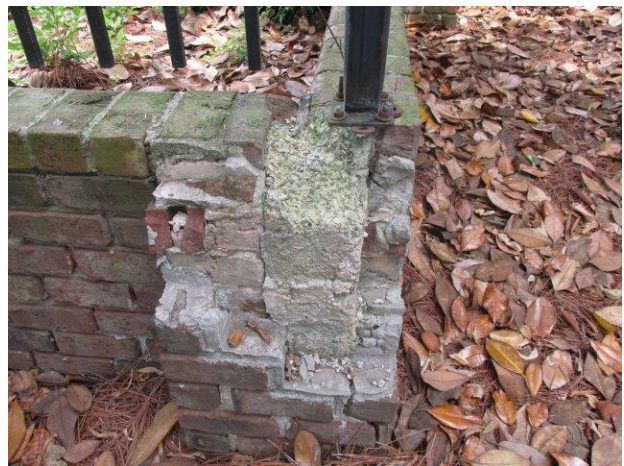
Damage to the masonry evident
