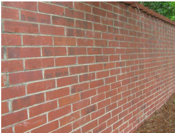
Perimeter wall overview
