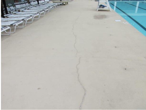
Concrete deck overview – previous crack repair evident
