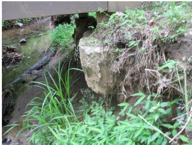
Exposed bridge footer due to erosion at the bridge
