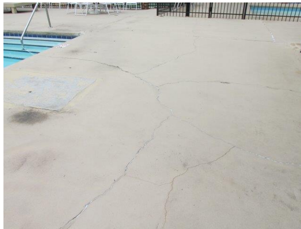
Concrete deck overview – surface cracks evident
