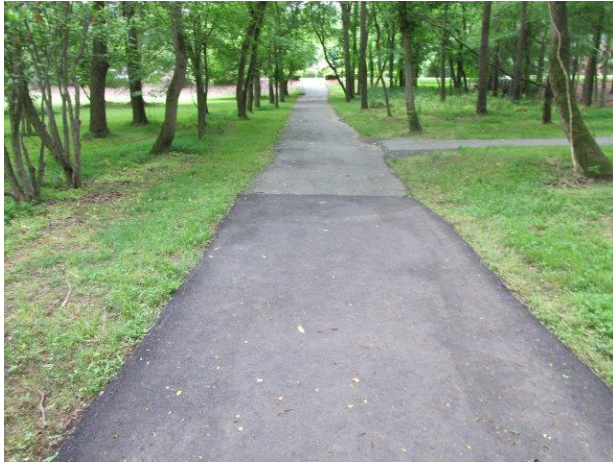
Overview of walking path – replacements evident
