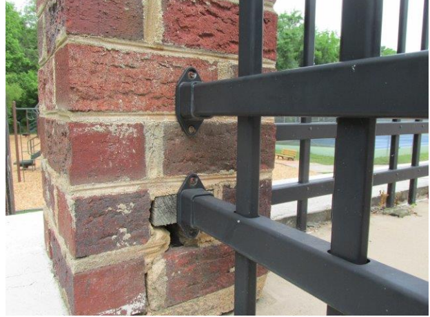
Masonry deterioration at column
