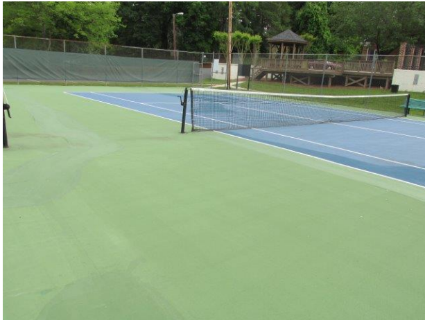
Tennis court overview
