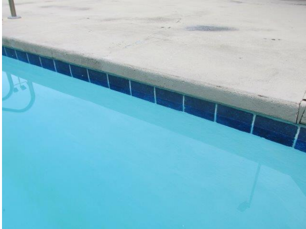
Plaster and tile at pool perimeter
