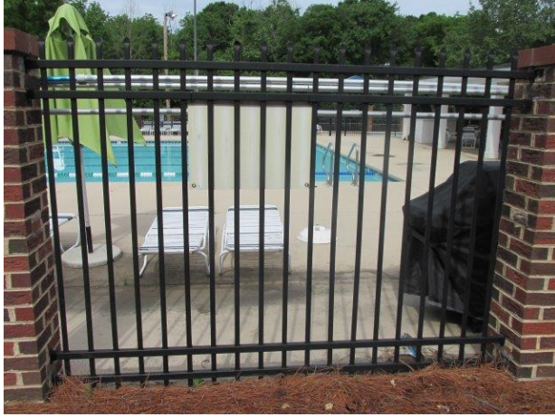
Aluminum fence at pool perimeter
