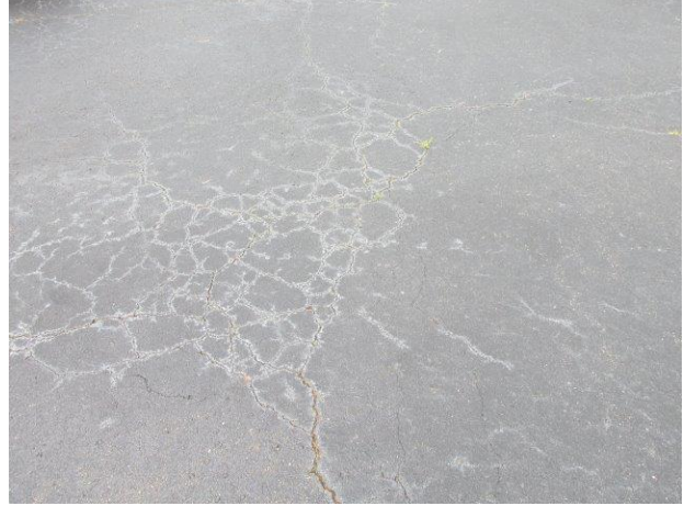
Example of alligator cracks
