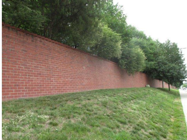
Perimeter wall overview
