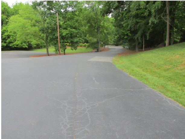
Asphalt pavement overview – surface cracks evident
