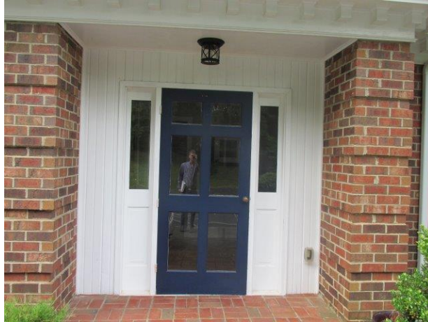
Front entrance at pool house
