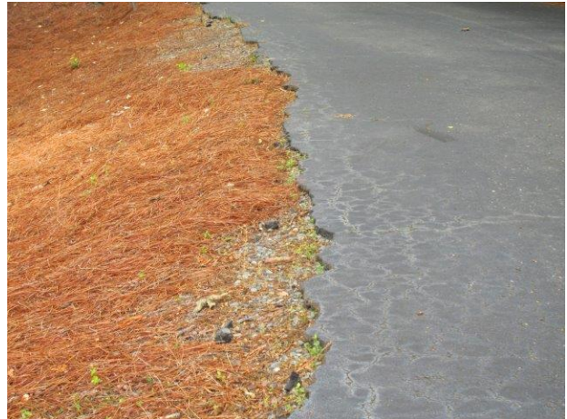
Deteriorated pavement at edge of parking lot
