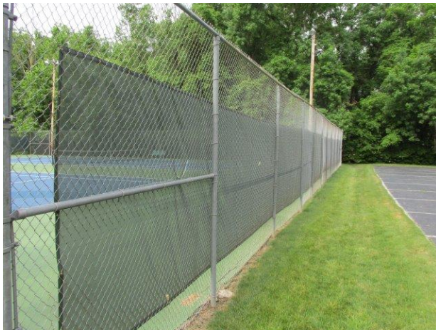
Chain link fence overview
