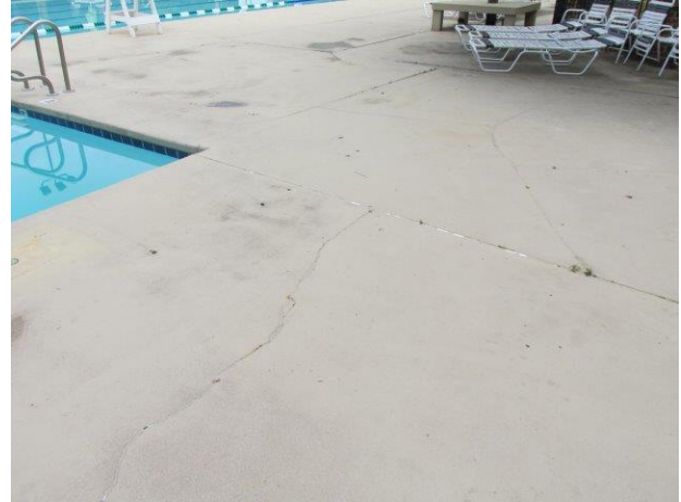
Concrete deck overview – surface cracks evident
