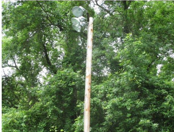
Typical light pole and fixture
