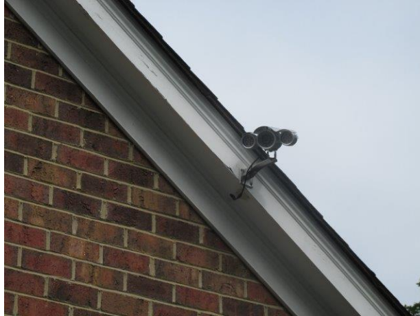
Example of typical security camera at the pool house
