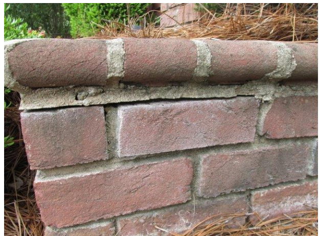
Mortar deterioration evident
