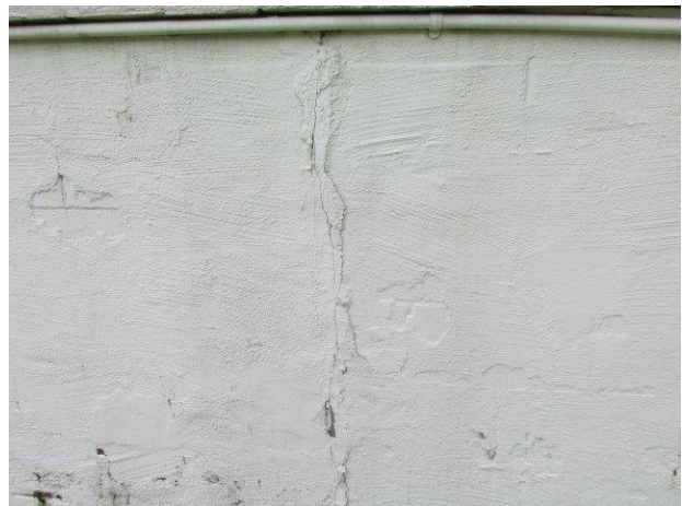
Cracks evident at retaining wall
