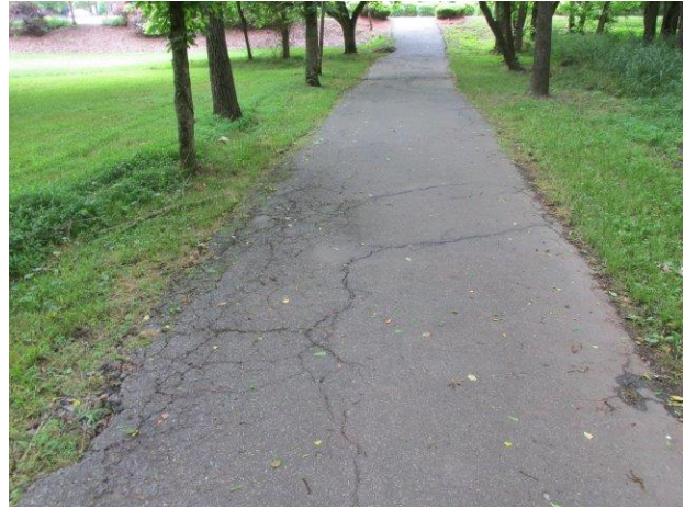
Walking path overview- surface cracks and deterioration evident
