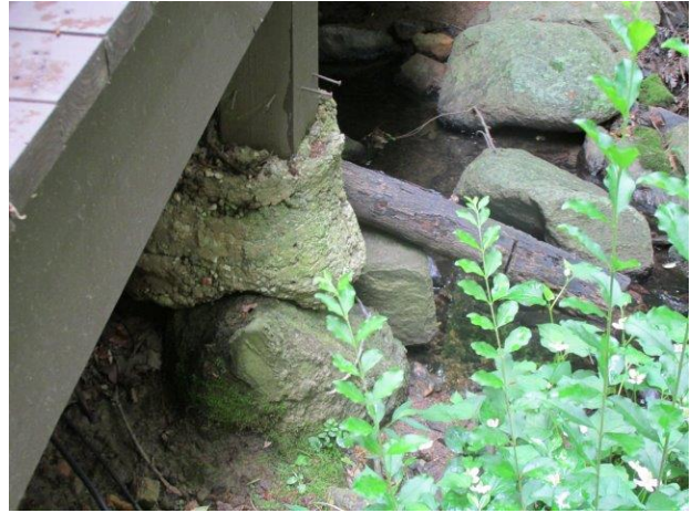
Area that has been washed out by the stream at the footer
