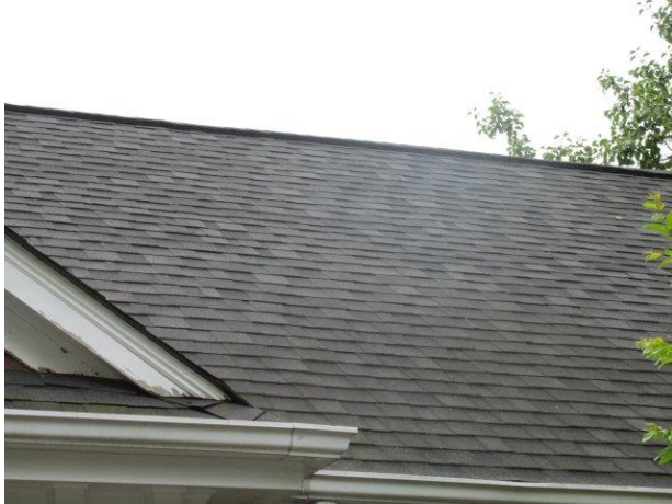
Asphalt shingle roof overview
