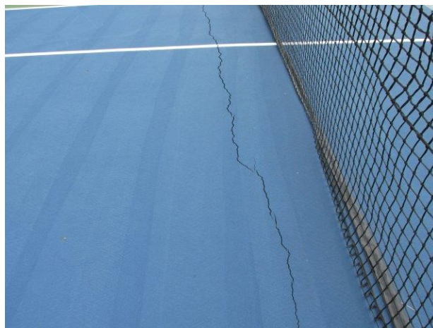
Surface cracks evident
