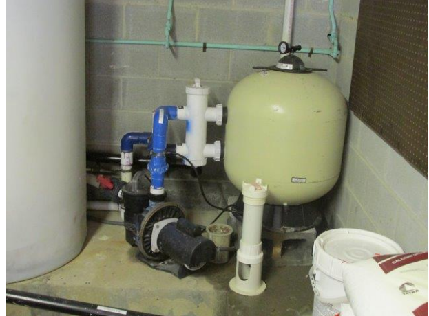
Spa pump and filter
