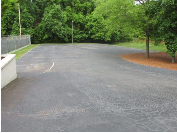
Asphalt pavement overview – alligator cracks evident
