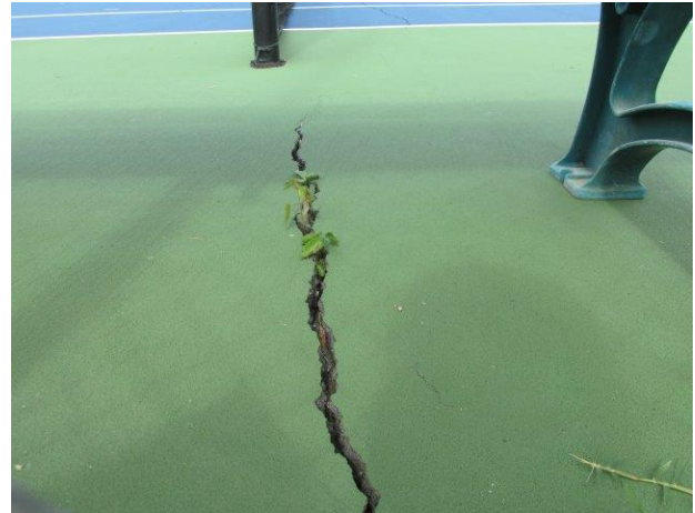
Surface cracks evident
