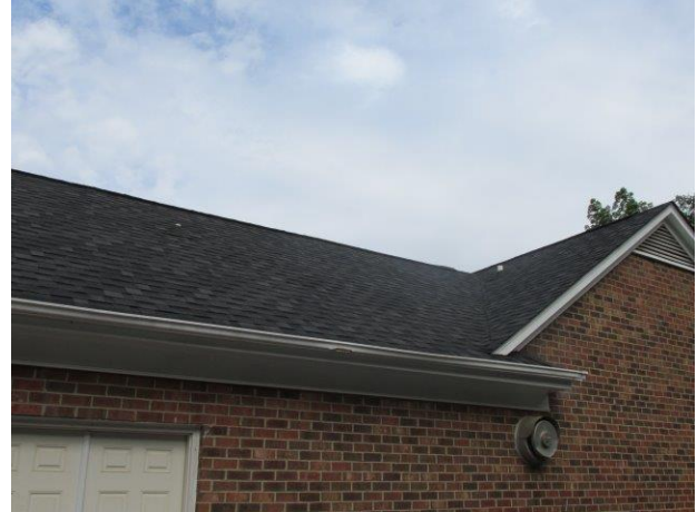
Enclosed full weaved valleys at asphalt shingle roof
