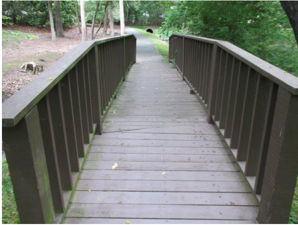
Overview of typical wood bridge
