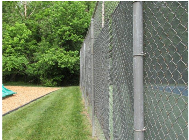
Chain link fence overview
