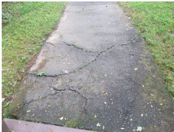
Surface cracks at walking path
