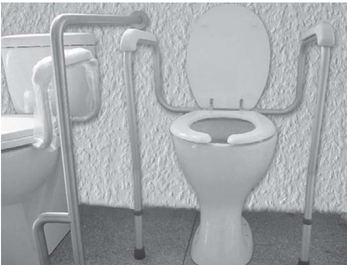
Figure 10.6: Grabrails in the bathroom and at the water closet
