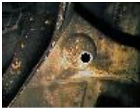
Figure 2: Predrilled counter-sink hole for bracket
