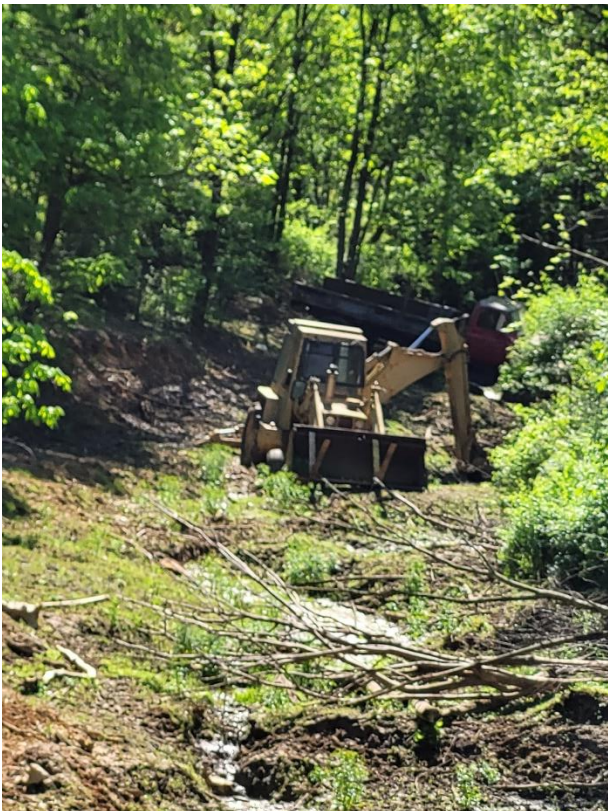
Picture 47 – Backhoe and farm truck The backhoe is being used to clear a waterway area that the PVC pipe in picture 46 will be used to divert water.
