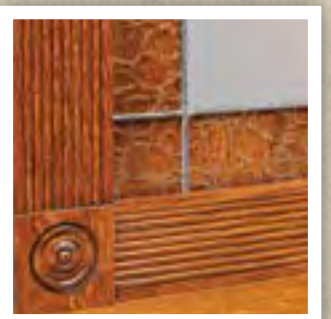
Cracked glass feature around mirror
