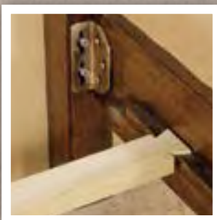
Rail and Slat Dovetail Construction
