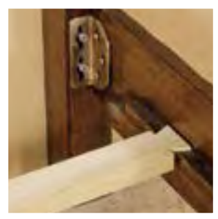
Rail and Slat Dovetail Construction
