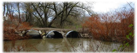
Multiple cross pipes on the Stillwater Creek crossing on Stoddard Road proved to be an issue and eventually led to increased flooding. The failing pipes eventually had to be partially removed and the road closed to the public.
