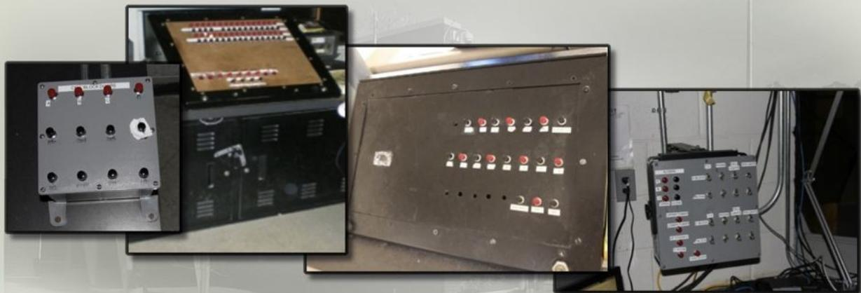
NON-ORIGINAL PANELS MAY CONTRIBUTE TO "GHOSTING" DOOR CONTROL ISSUES, WHICH ARE KNOWN TO UNLOCK DOORS THROUGHOUT THE FACILITY ON A RANDOM BASIS. AS A RESULT, EMERGENCY FIRE EXIT DOORS HAVE BEEN DISCONNECTED FROM THE DOOR CONTROL SYSTEM AND POSE A SUBSTANTIAL LIABILITY FOR THE COUNTY.
