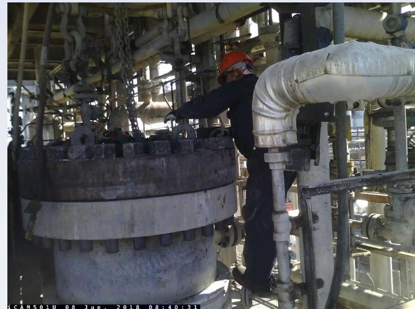
There have been many problems with the DMJ gaskets sealing even though a full written procedure is in place and the bolt to gasket stress checks out in theory. Seal ability had become a major cost issue due to the inconsistency and down time of the reactors. Leakage was occurring on both the top and bottom flanges of the poly reactors.
