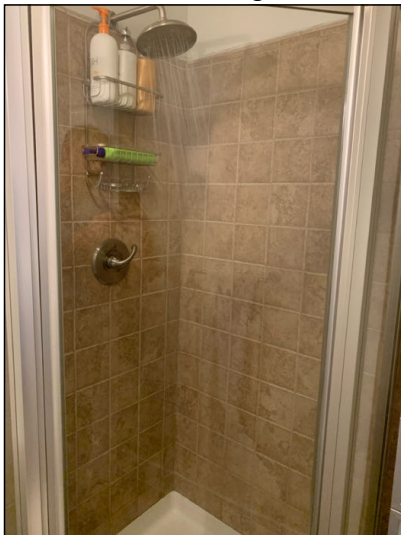
Main level Bathroom
