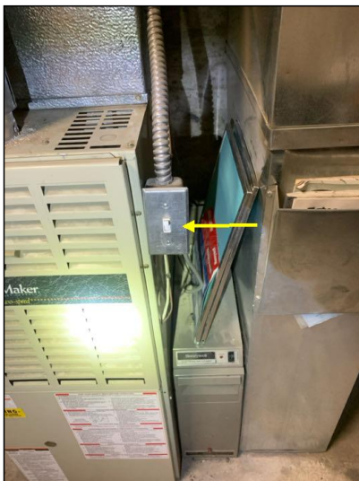
Main turn off switch for the Heater HVAC system.
