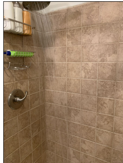
Main level Bathroom
