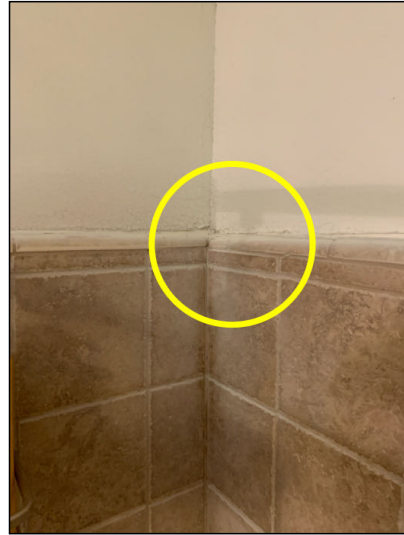
Main level Bathroom
