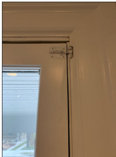
This window is operational, the latching mechanism is painted so it doesn't open properly.
