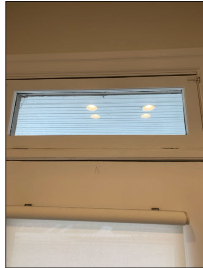
This window is operational, the latching mechanism is painted so it doesn't open properly.
