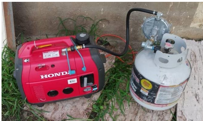
Fig. 3. Converted Honda EU2200i generator and propane tank deployed in Haiti (May 2023)
