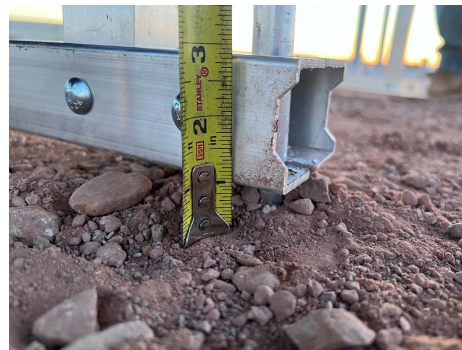
PHOTO 5: Ground to frame measurement example at Spike #3
