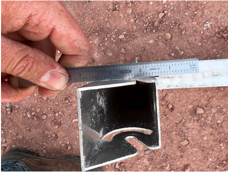
PHOTO 11: Slight deformation after load removed
