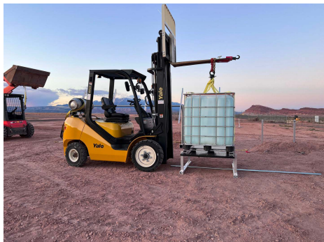
PHOTO 4: Setting initial load
