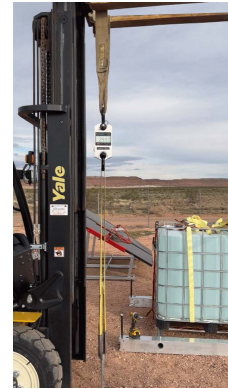
PHOTO 3: Second anchor under load
