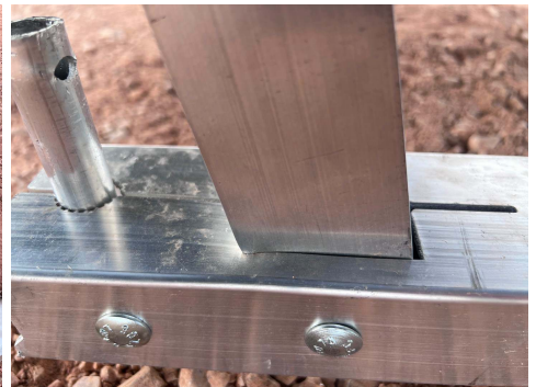
PHOTO 15: Upright deformation after testing
