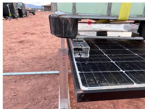
PHOTO 8: Slight deflection noted under load
