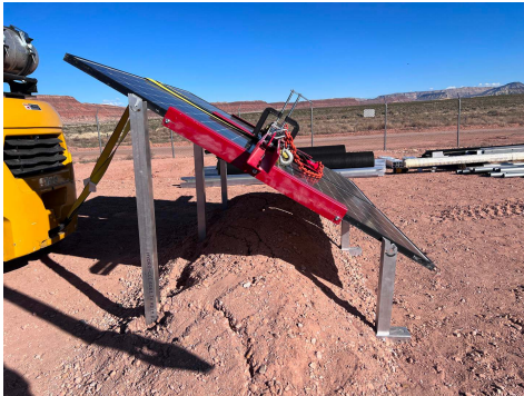
PHOTO 13: Ballast after completion of testing
