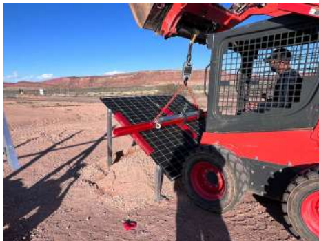
PHOTO 4: Test setup with dynamometer and chains connected
