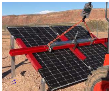
PHOTO 8: Test 2 - Evidence of ballast shift
