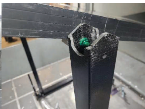
Figure 17: IR Ballast frame connection to solar panel
