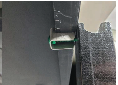
Figure 18: IR Ballast frame connection to solar panel
