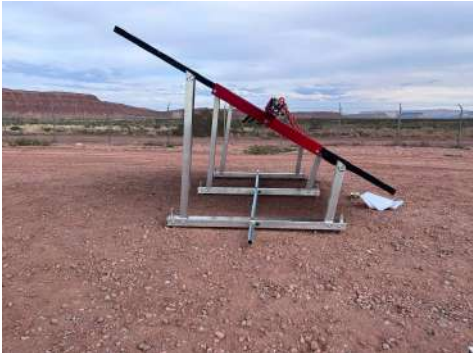
PHOTO 11: Frame after testing
