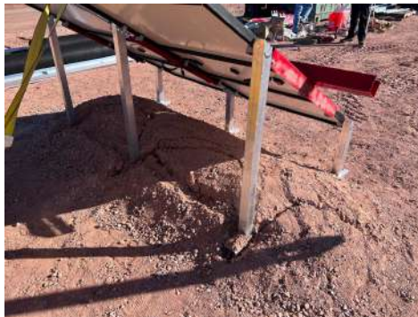
PHOTO 14: Ballast and frame after completion of testing
