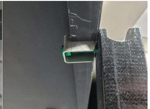
Figure 18: IR Ballast frame connection to solar panel
