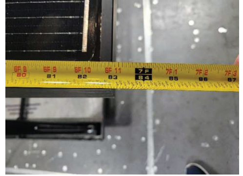
Figure 21: Solar panels total length 83 in.
