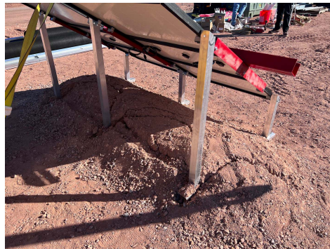
PHOTO 14: Ballast and frame after completion of testing
