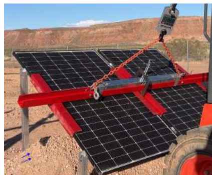
PHOTO 8: Test 2 - Evidence of ballast shift
