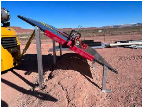
PHOTO 13: Ballast after completion of testing
