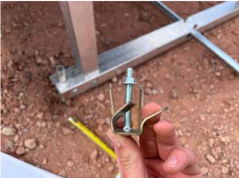
PHOTO 13: Bracket deformation after testing
