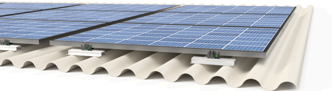
Asbestos / Cement Board Roofs
