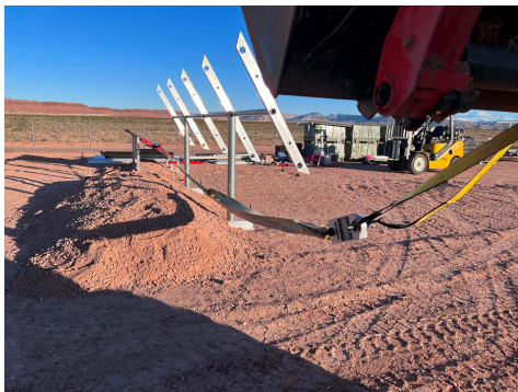
PHOTO 3: Horizontal force test setup
