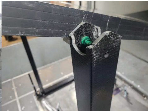
Figure 17: IR Ballast frame connection to solar panel
